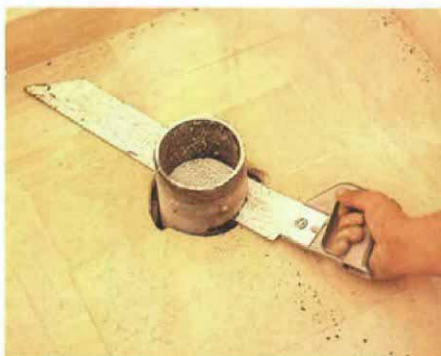
2. Before installing a closet flange, cut the plastic pipe flush with the floor.
