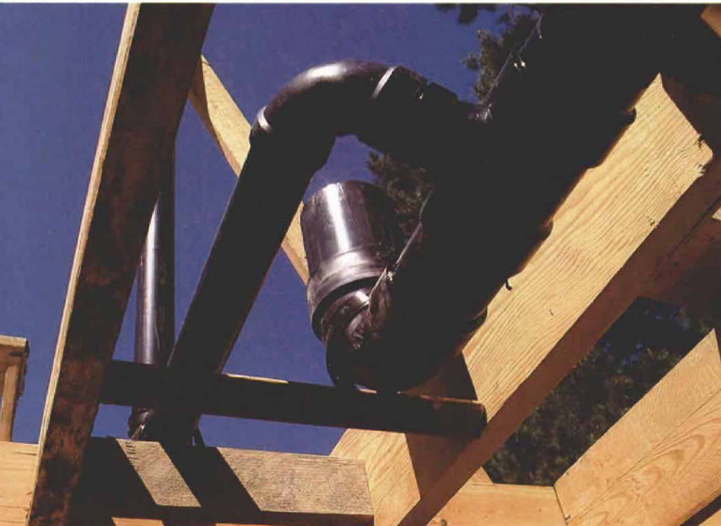
1. In wood-frame construction, a closet bend should be supported from below with a 2x4 block and held in place with strapping.
