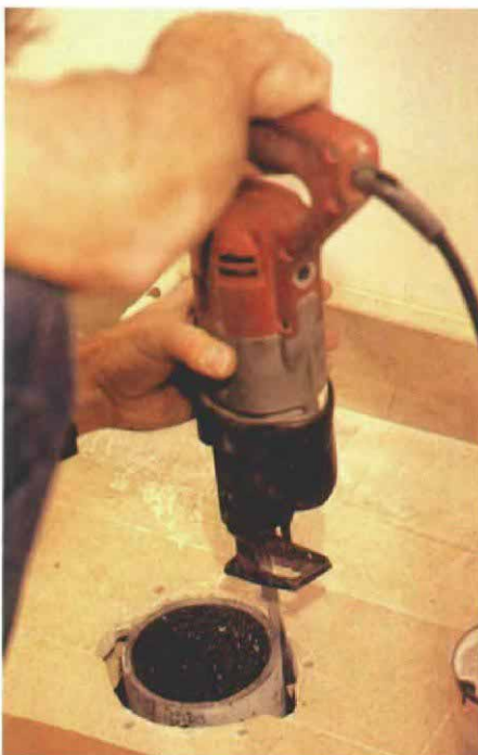
4. Sometimes tile or stone floor coverings will crowd the pipe stub, making it difficult to install the closet flange. When this happens, use a cold chisel or a reciprocating saw to make room for the flange.
