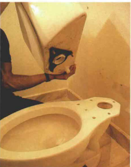
12. Two-piece, or close-coupled, toilets have separate bowls and tanks that must be bolted together carefully.
